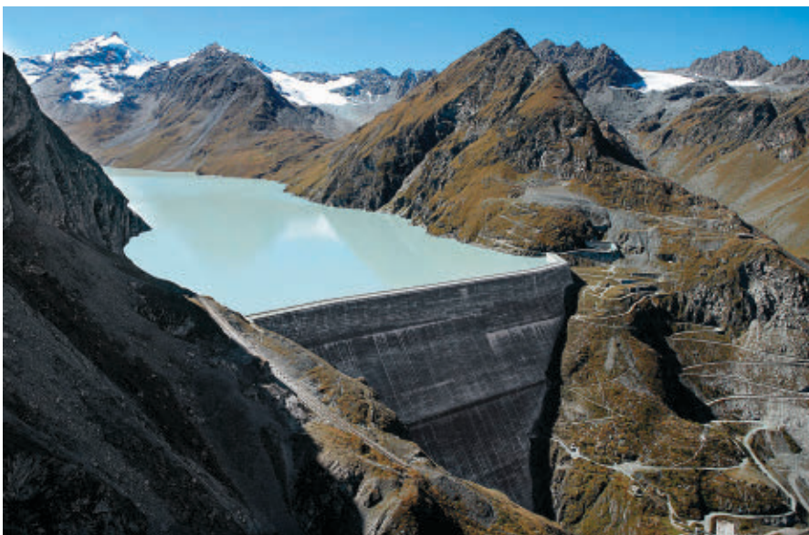
Figure 14. Grande Dixence in the Swiss Alps, the world's highest concrete dam, relied on calculations aided by the Zuse Z4 and electromechanical desktop calculators (such as Madas from H. W. Egli AG, Zürich-Wollishofen). Courtesy of Grande Dixence SA, Sion, Switzerland.
