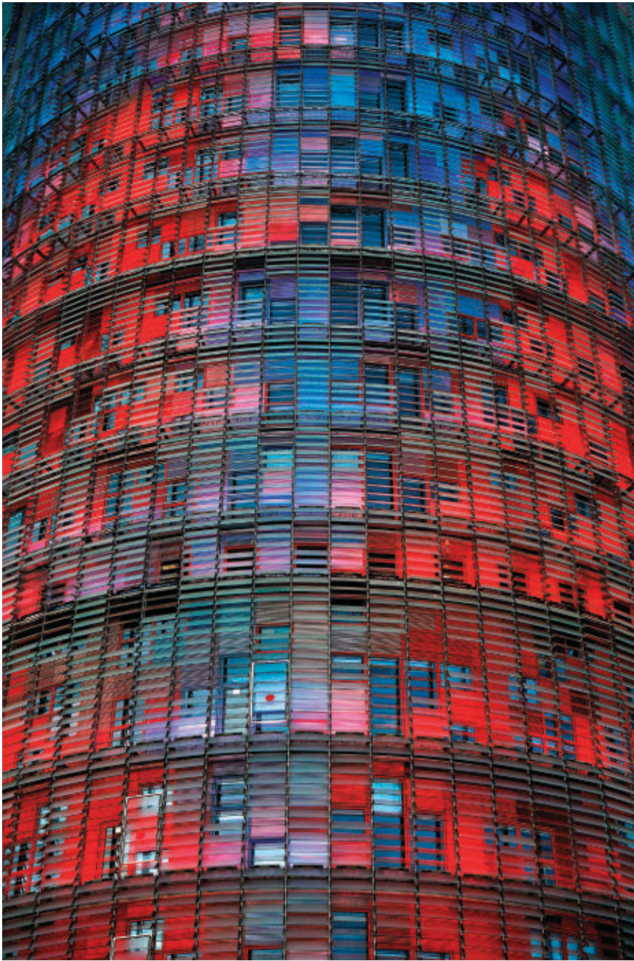
Torre Agbar (Agbar Tower) in Barcelona is covered with more than 4,500 luminous devices capable of creating 16 million colors.
