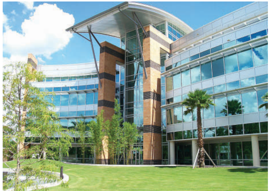
The Harris Engineering Center, home of the School of Electrical Engineering and Computer Science at the University of Central Florida, USA.
