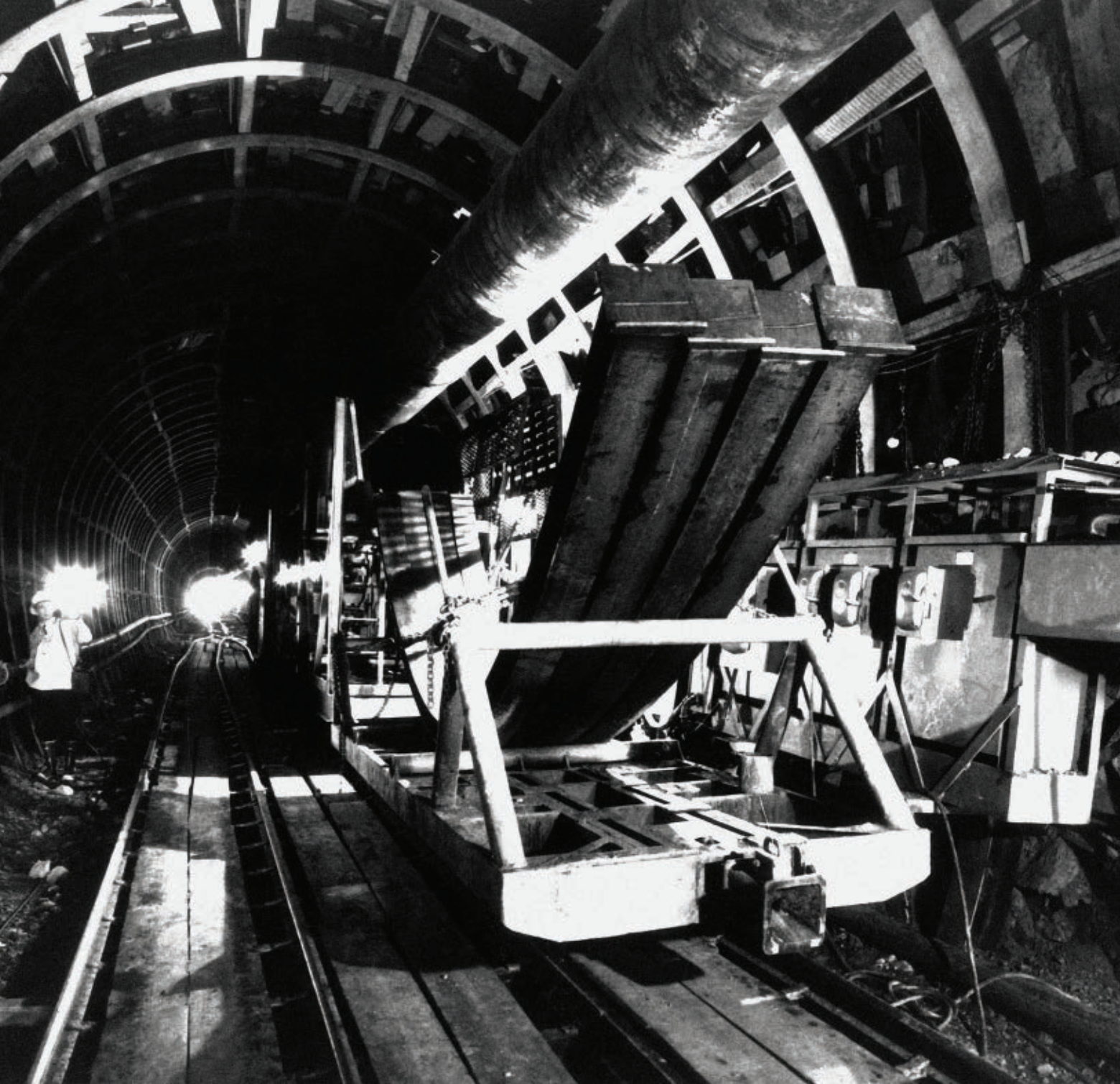
The Transbay Tube during its construction in the 1960s.
