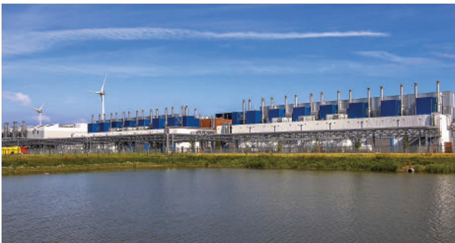
Google’s datacenter in Eemshaven, Netherlands, has been powered entirely by renewable energy since the day it opened in late 2016.
